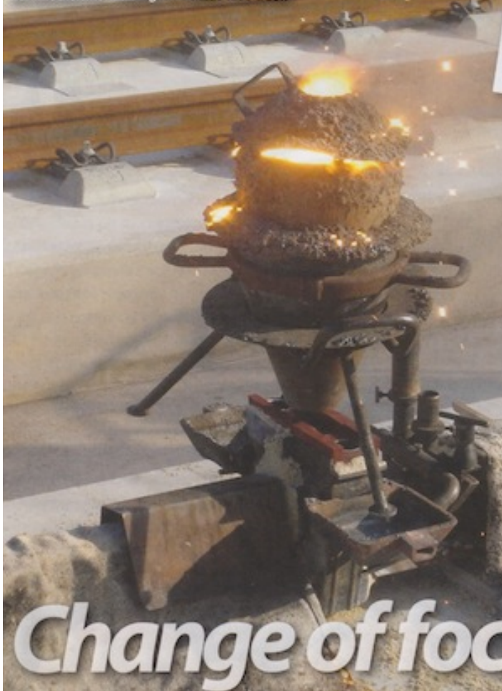
Aluminothermic welding on ballast-less track
