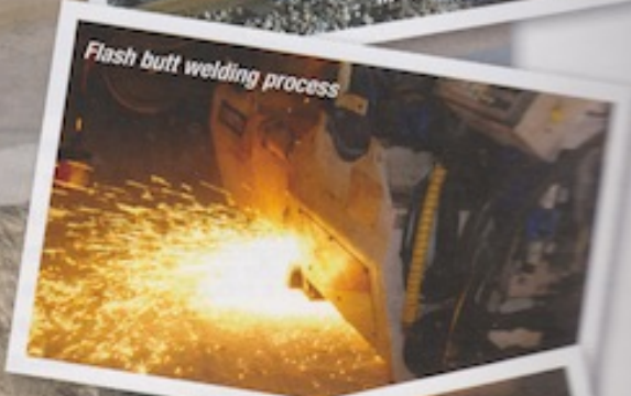
In situ flash butt welding
