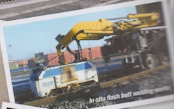
Flash butt welding process
